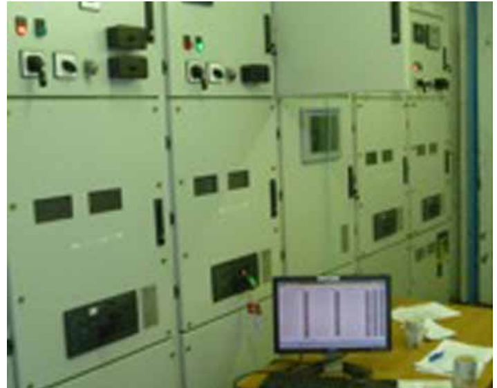
New MCC During Commissioning
