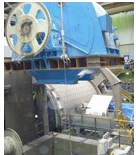
3200KW SAG Mill Motor being lowered into position
