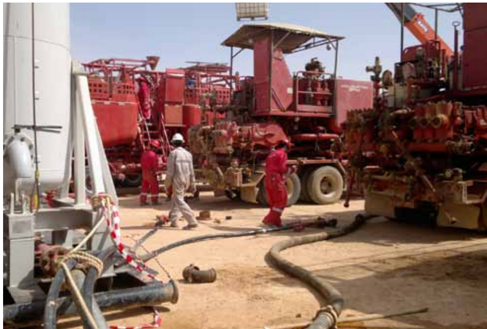
HDPE pipes cement job in progress
