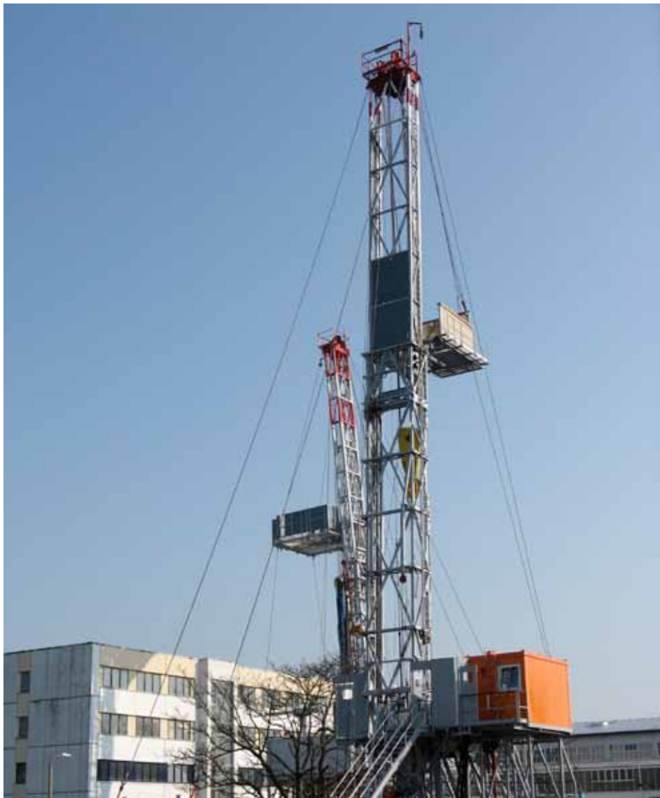
Rig 45 at SATVIA yard
