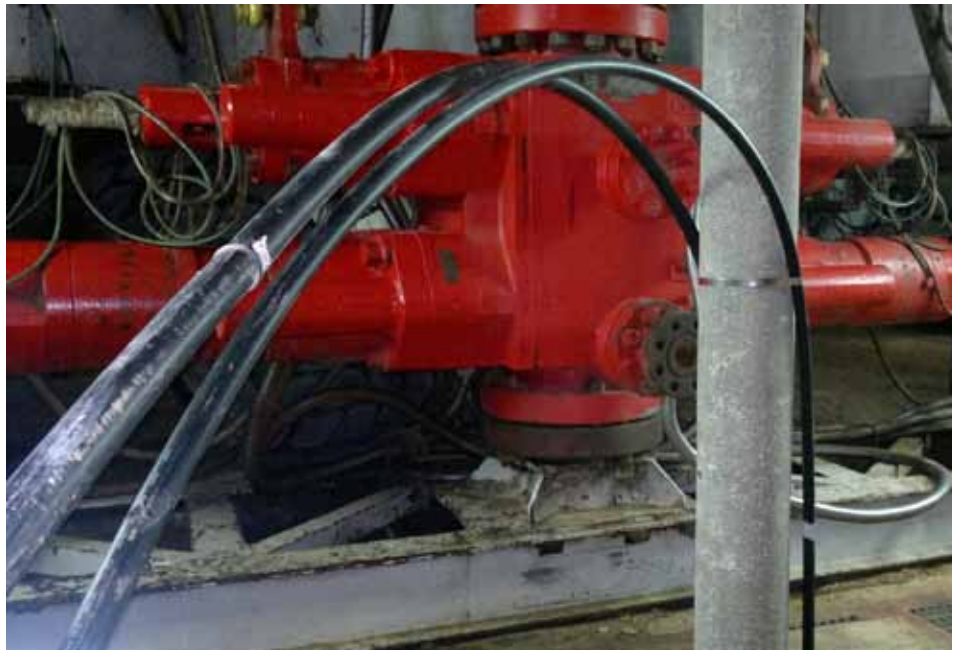
Strapped HDPE pipes while the casing is run in
