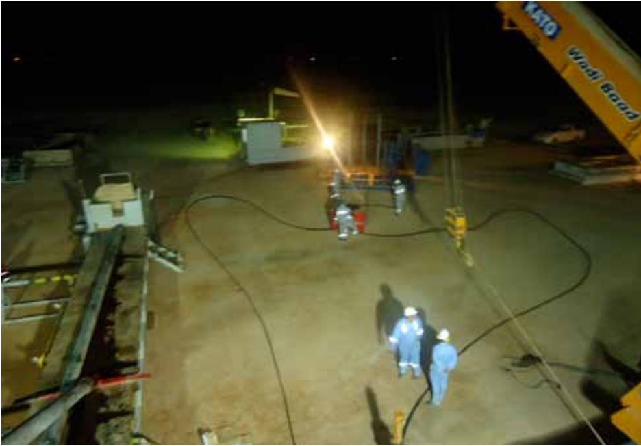
Slagged HDPE pipes being fed to the casing for strapping
