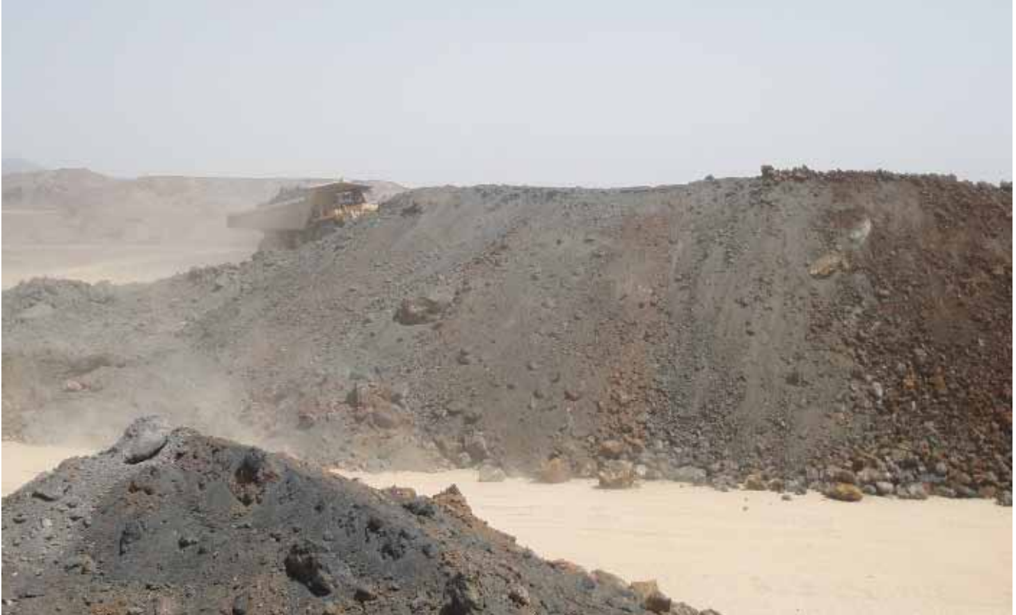
Another 40 tonnes of Copper ore.....A CAT 771 dump truck with an approximately 40 tonne payload makes its way up the ore stockpile dump. By end of May 2011 over 70 000 tonnes of Transitional Zone Copper ore had been mined and stockpiled at Safwa
