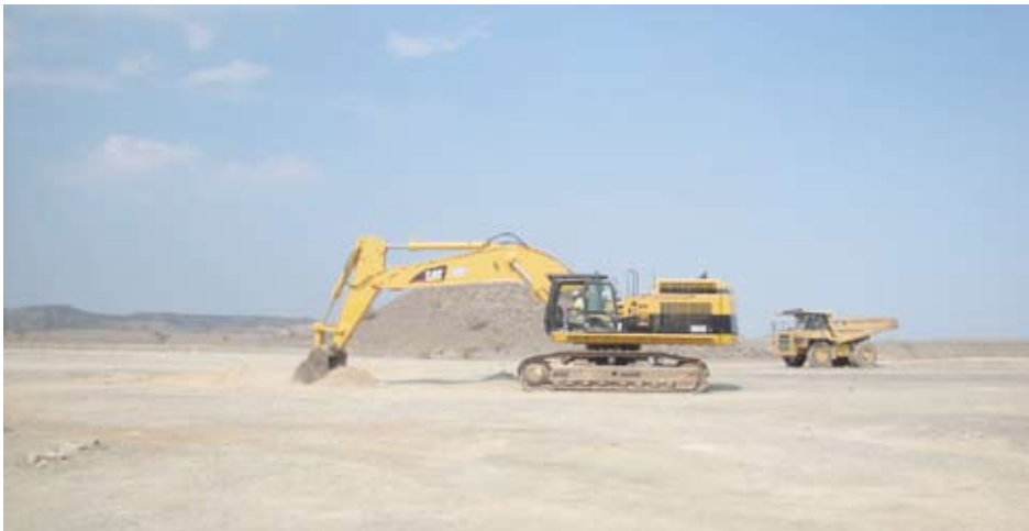
Commencement of excavation works October 31st 2010
