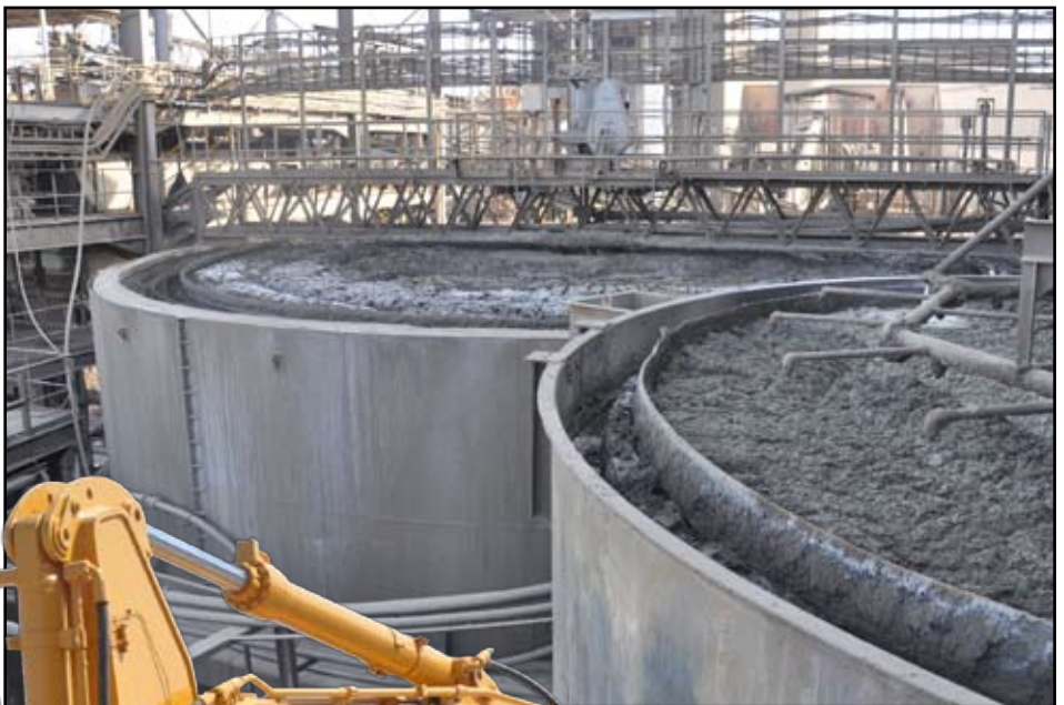
Copper extraction operation at Lasail plant
