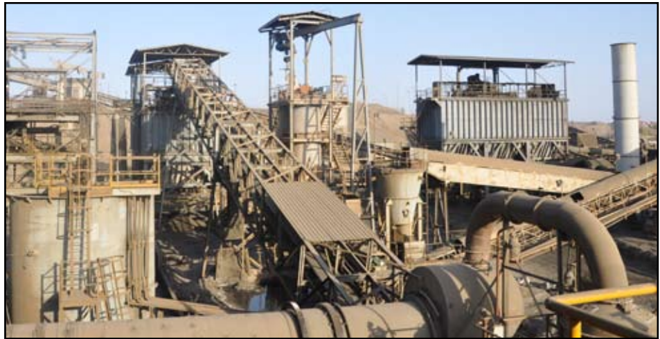
Lasail plant in Sohar
