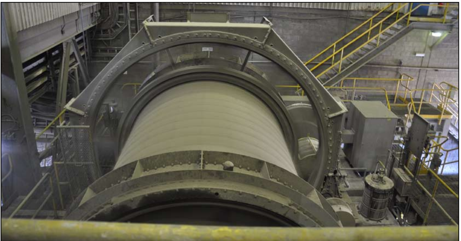
SAG mill in Lasail plant
