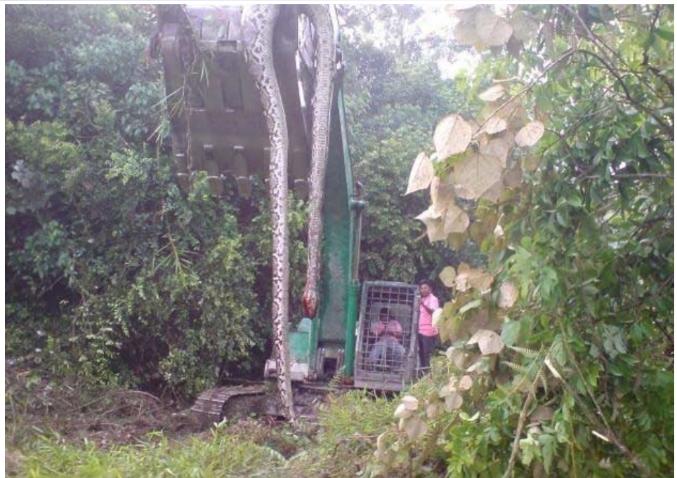
A snake captured by the construction crew while building the ASAP .1 location at Nagote, West Papua. The snake, believed to be a Reticulated Python was about 13 metres long and it had a wild pig inside it that weighed approximately 150 kg.
