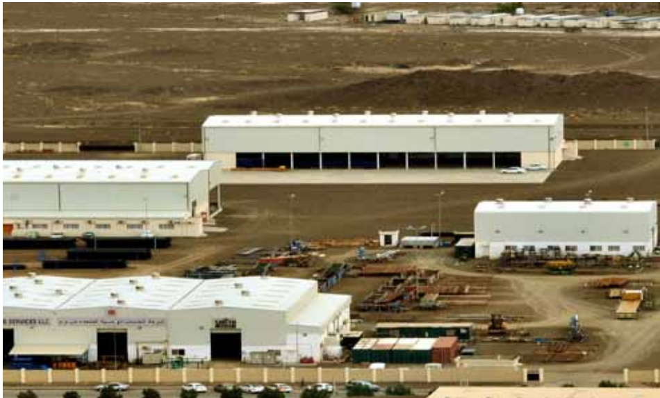
The UES facility in Nizwa
